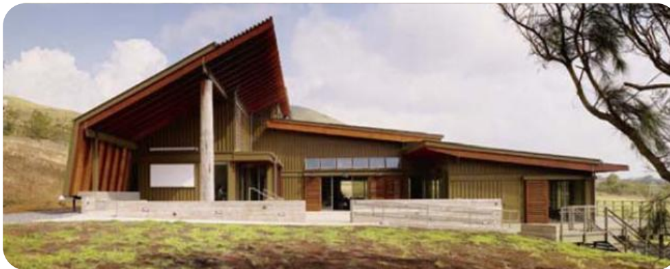
The Energy Lab, Kamuela Hawaii
